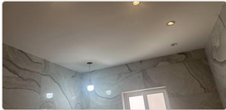
A43 SITE: main bathroom — ceiling & downlights [BTH]
