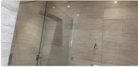
A37 SITE: ensuite — existing shower enclosure [ENS]
