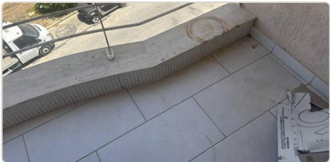
A06 SITE: front balcony — already tiled, membrane at edge [FBL]
