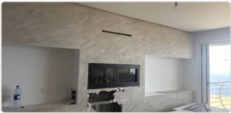
A17 SITE: dining feature wall + fireplace, wall opened below [OPN]
