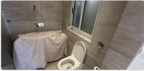
A39 SITE: ensuite — WC & window [ENS]
