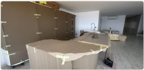
A16 SITE: kitchen island, units wrapped [OPN]
