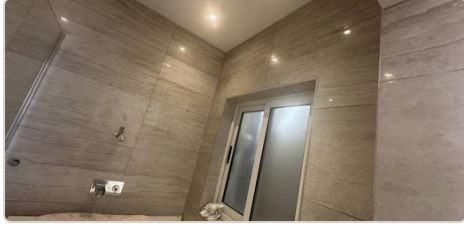
A40 SITE: ensuite — overview [ENS]
