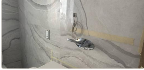
A41 SITE: main bathroom — existing finish [BTH]
